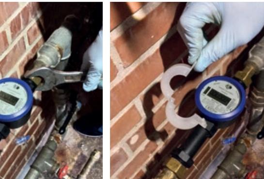
A technician from Tårnby Forsyning in the process of replacing a mechanical meter with a remotely read meter.
